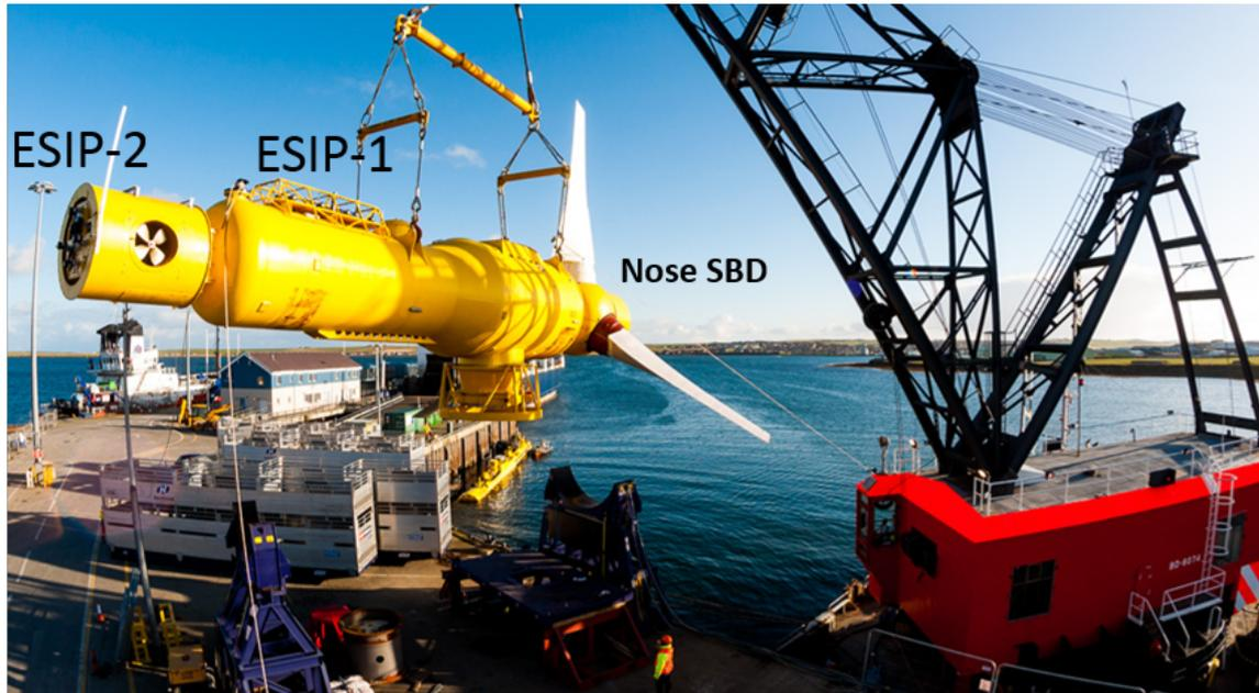
Figure 1: Photograph of DEEPGEN IV being lifted by crane barge prior to deployment. Locations of the UoE instrument platforms, ESIP-1, ESIP-2 and the nose SBD identified.
