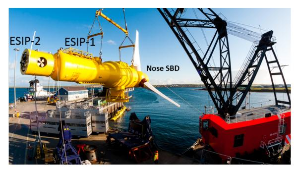
Figure 1: Photograph of DEEPGEN IV being lifted by crane barge prior to deployment. Locations of the UoE instrument platforms, ESIP-1, ESIP-2 and the nose SBD identified.
